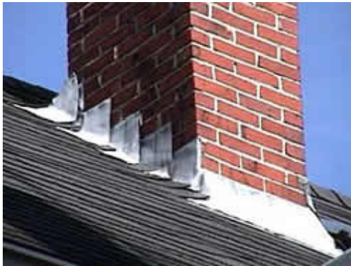
Protect and maintain a roof by cleaning the gutters and downspouts and replacing deteriorated flashing. -- http://www.cr.nps.gov/hps/tps/standguide/rehab/rehab_roofs.htm
