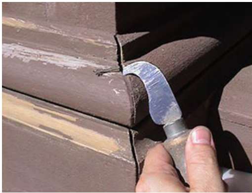
Cracks and unpainted wood on porch elements can lead to decay due to water seepage. Proper caulking and painting can help preserve these elements. -- http://www.nps.gov/tps/how-to-preserve/briefs/45-wooden-porches.htm
