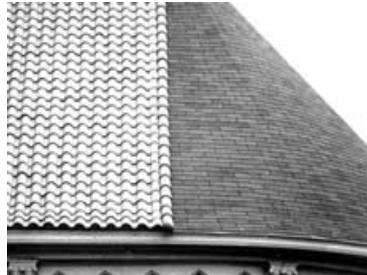
Asphalt shingles are an incompatible replacement substitute for the original Spanish clay tiles. -- http://www.cr.nps.gov/hps/tps/standguide/rehab/rehab_roofs.htm
