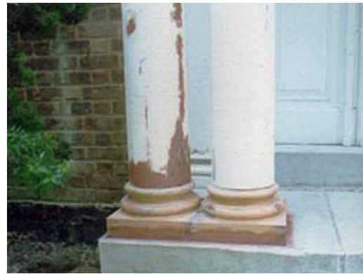
Deteriorated wood porch elements can be repaired in place with epoxy consolidants and fillers. -- http://www.nps.gov/tps/how-to-preserve/briefs/45-wooden-porches.htm
